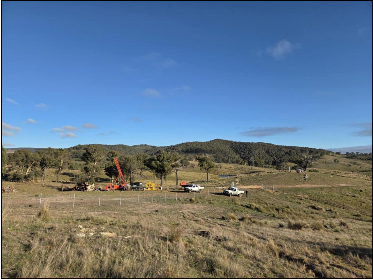
Figure 5: Drill rig set up at the Picker Prospect.
